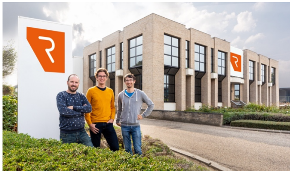
REIN4CED's new automated bicycle frames production facility in Leuven, Belgium.
